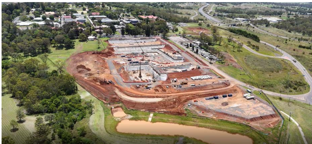
Figure 20: Baillie Henderson site works status February 2025
